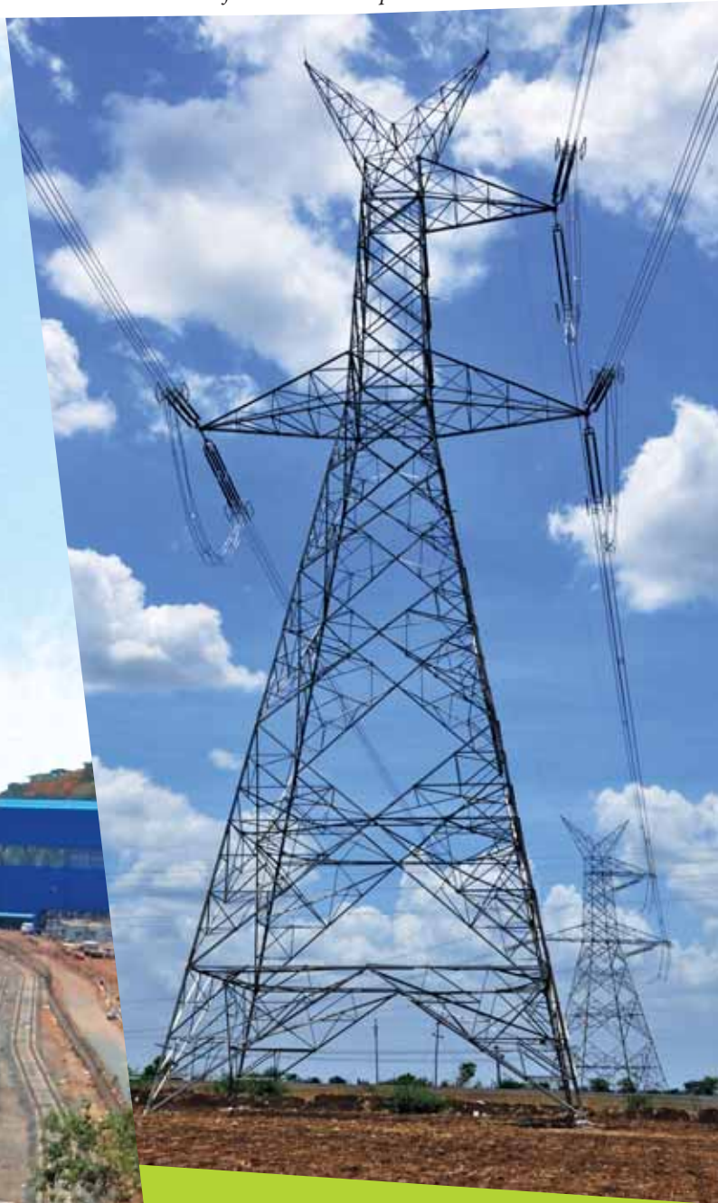
208 KM long Transmission line of 765KV Single Circuit for Raichur Sholapur Transmission Co. LTD
