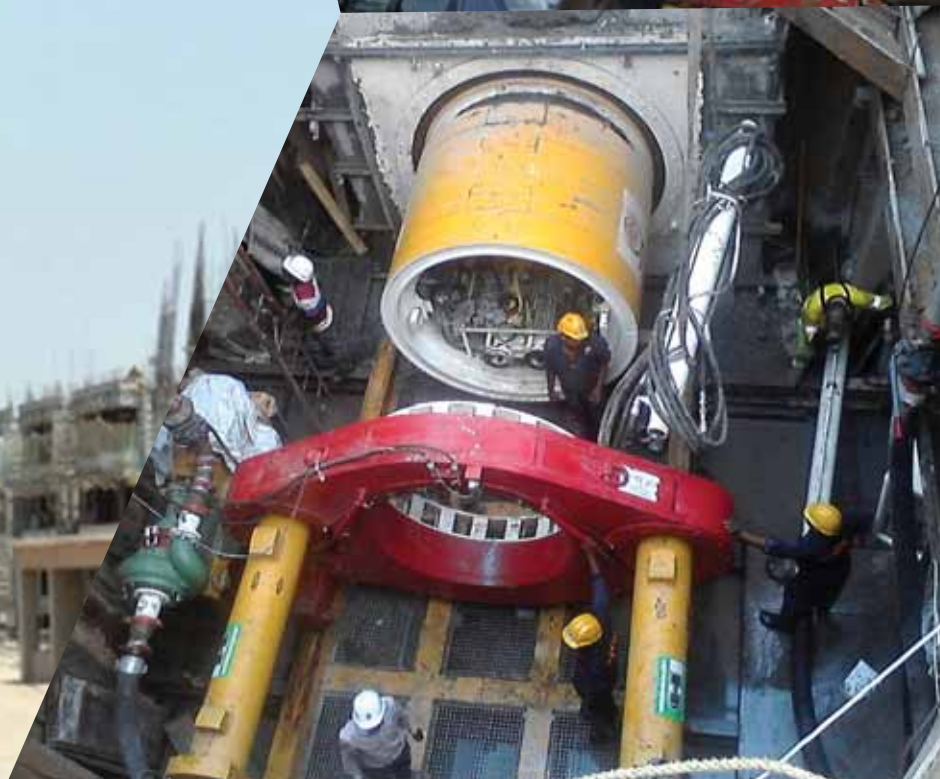
Micro tunneling work in progress for laying of 1829 mm dia concrete lined pipeline for water supply project at New Town, Kolkata
