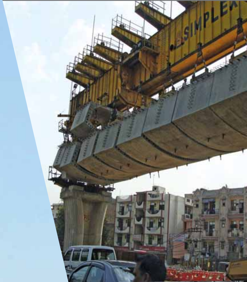
Precast Spine Lifting under progress for PWD Flyover work at Vikaspuri, New Delhi
