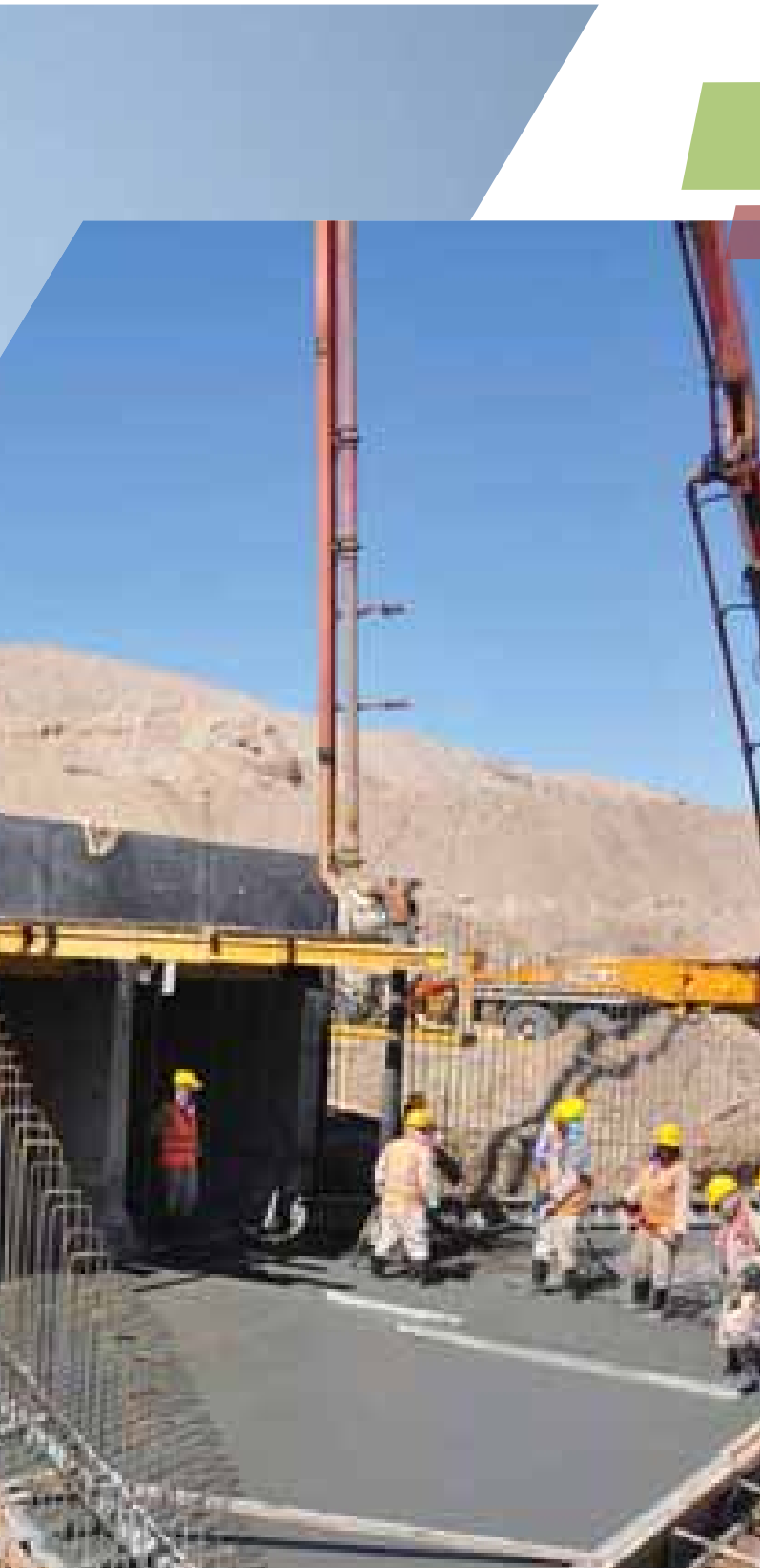
RCC Box Culvert work in progress
