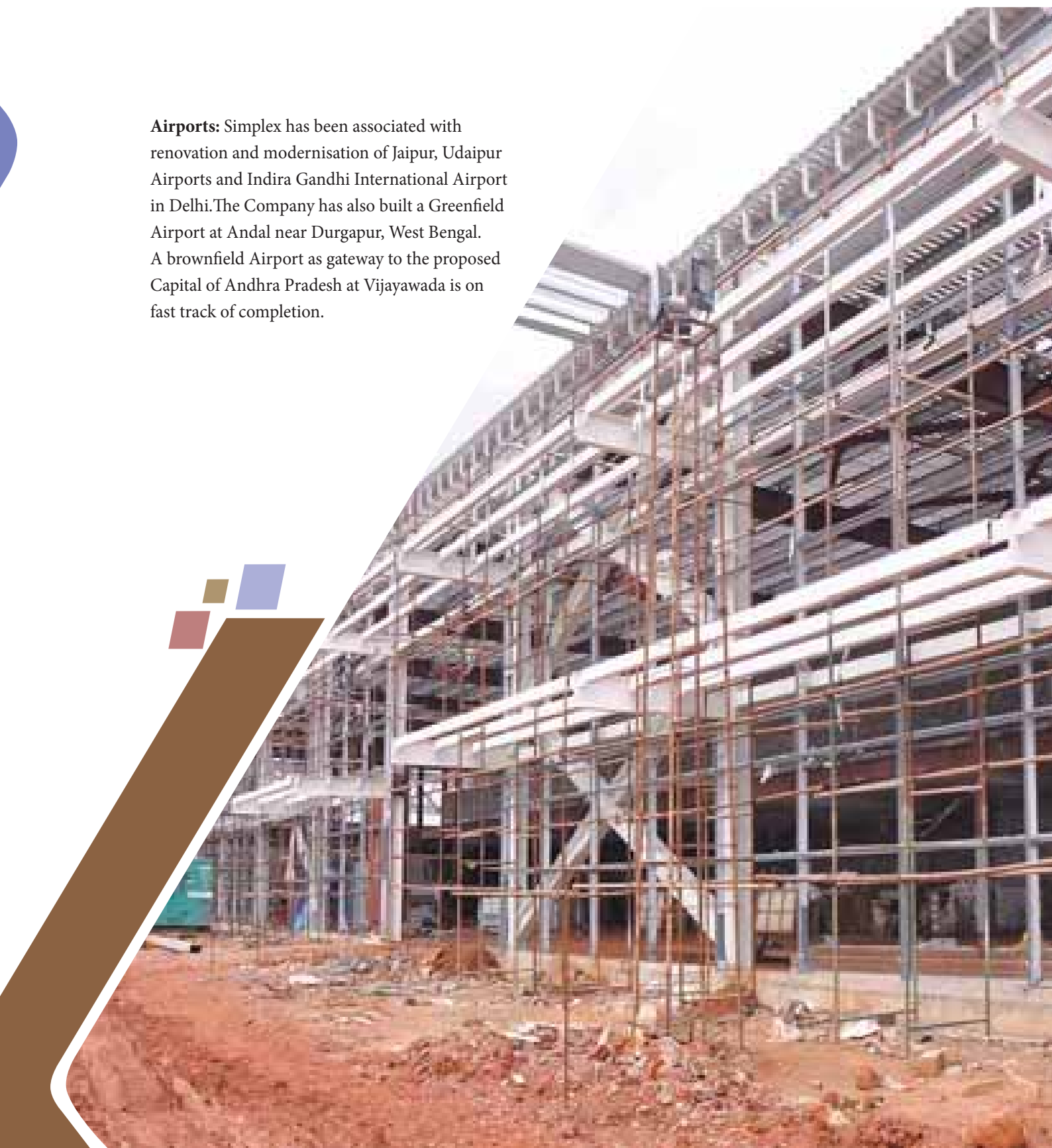
DGU Facade Frame over Structural Work for new Vijayawada Airport Terminal, Andhra Pradesh
