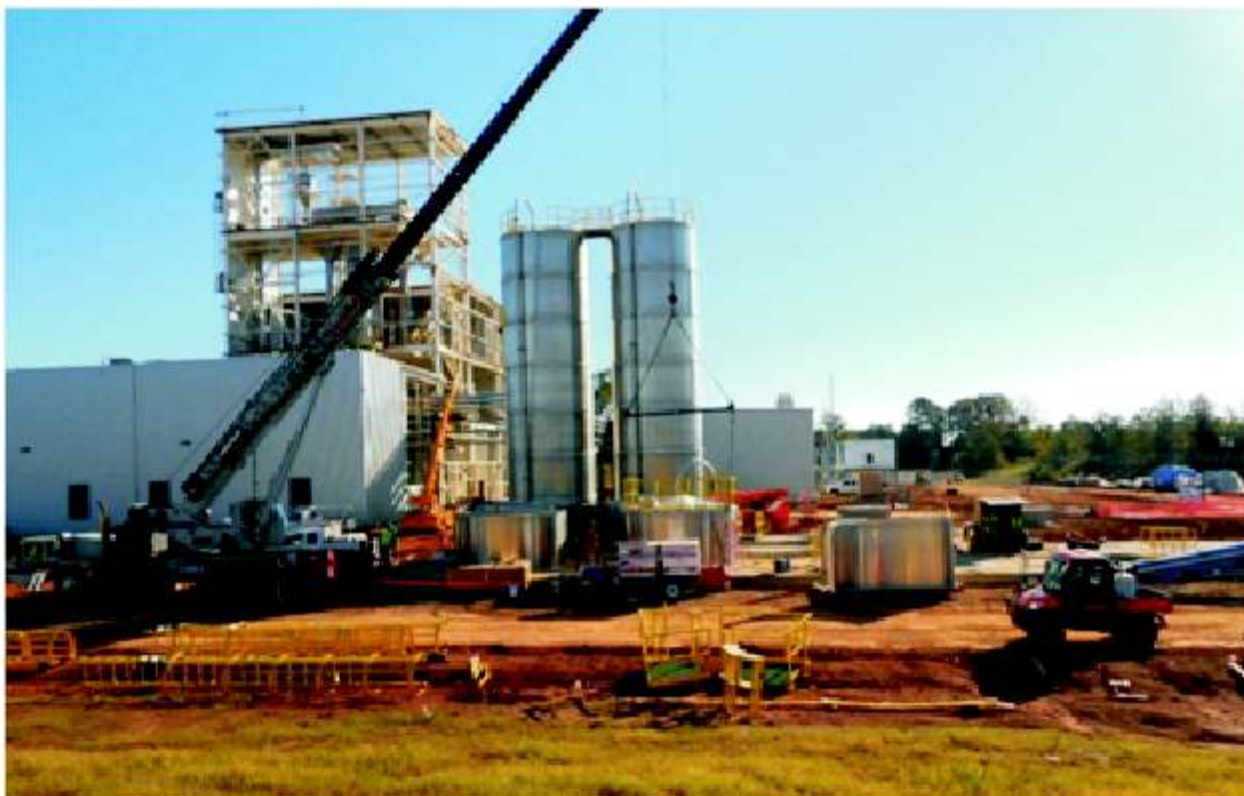
Resin Silo installation at Decatur, Alabama, USA
