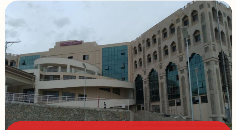
Hospital Project In Udaipur Rajasthan
