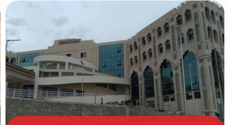
Hospital Project In Udaipur Rajasthan
