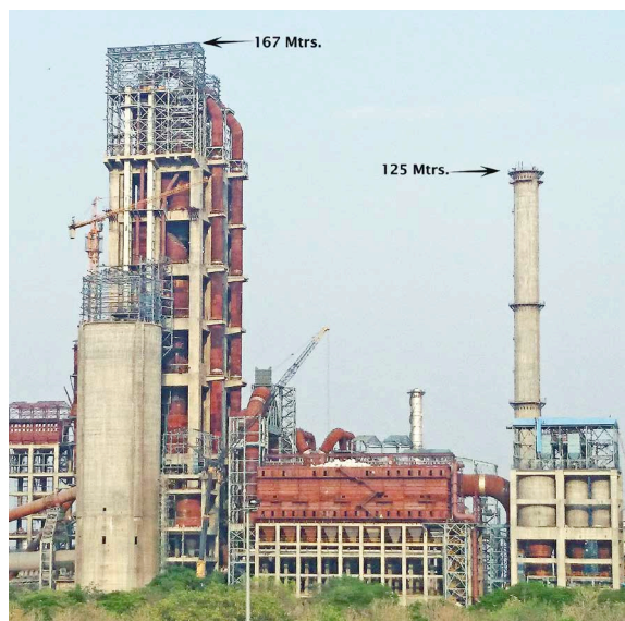
Manikgarh cement unit-II 2.8 Mtpa capacity under erection
