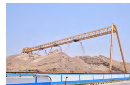
Raw Material Storage and Chipping
