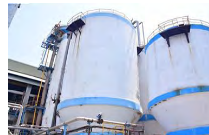
Fiber Line Pulp Mill
