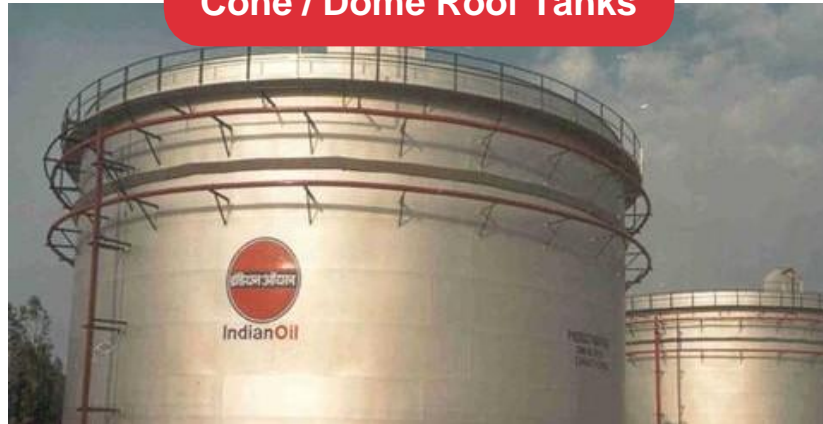
Cone / Dome Roof Tanks
