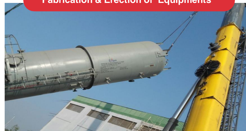
Fabrication & Erection of Equipments
