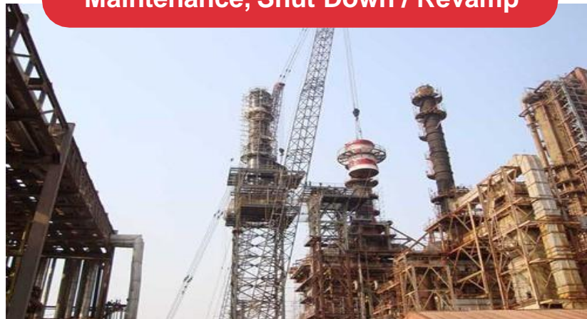
Maintenance, Shut Down / Revamp
