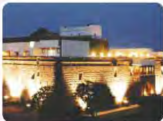
Fort Jadhav GADH A Green Heritage Hotel Ladh, Jhagadh, Aaga Badh... PUNE, MAHARASHTRA
