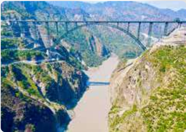
Chenab Railway Arch Bridge
