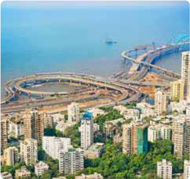
Mumbai Coastal Road Project (MCRP)
