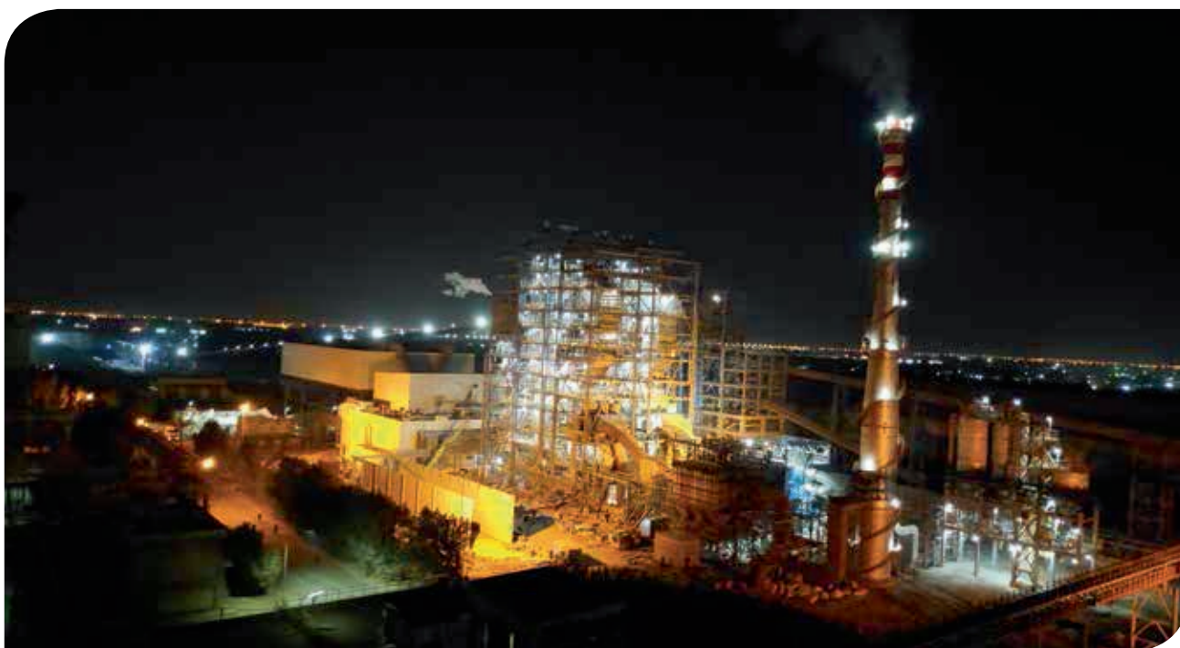
A 40 MW coal-based captive power plant commissioned for a leading cement and clinker manufacturer in the UAE. It comprises two CFBC boilers of 90 TPH capacity each that are capable of firing multiple varieties of coal along with a first-of-a-kind 30% wood chip firing.
