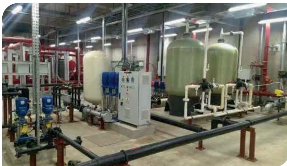
A Water Treatment Plant commissioned by Thermax for a Swedish furnishing major's first store in India. The plant produces 2,000 litres of treated water per hour, catering to the potable and non-potable water requirement of the entire store.
