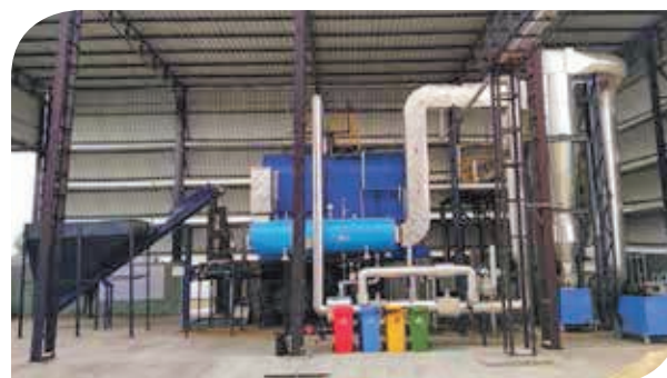
Combloc UFS 30, a 3 TPH boiler installed in Maharashtra for a German multinational producing animal feed. This biomass fuel-based boiler is semi-automatic, designed for small-sized plants.
