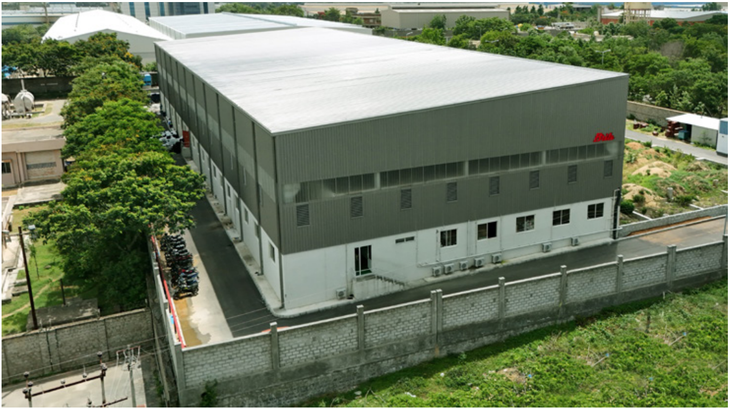
Manufacturing facility at Hosur in 2023
