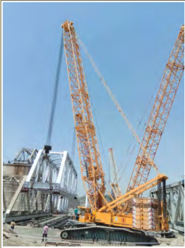
Liebherr LR 1400/2 and TerexDemag CC 2400-1 (400 MT crawler crane) working in Gujarat for the installation of railway bridge across the Mahi river.
