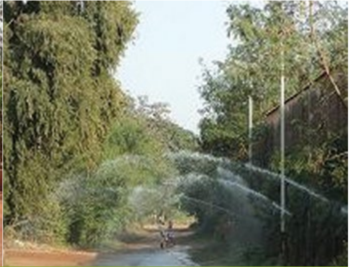
Dust Suppression System by Using STP treated water
