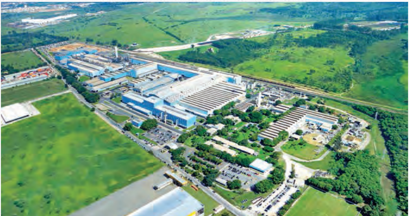
Novelis' recycling plant in Pinda, Brazil
