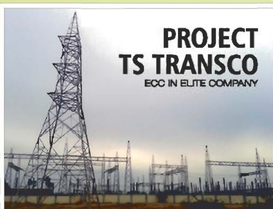
55 meter high HMD Transmission Towers for 220 KV Sub-Station & Transmission Line has earned the distinction of erecting the highest tower.
