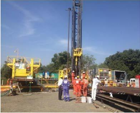
CBM Production Drilling At Sohagpur, MP For Reliance Industries
