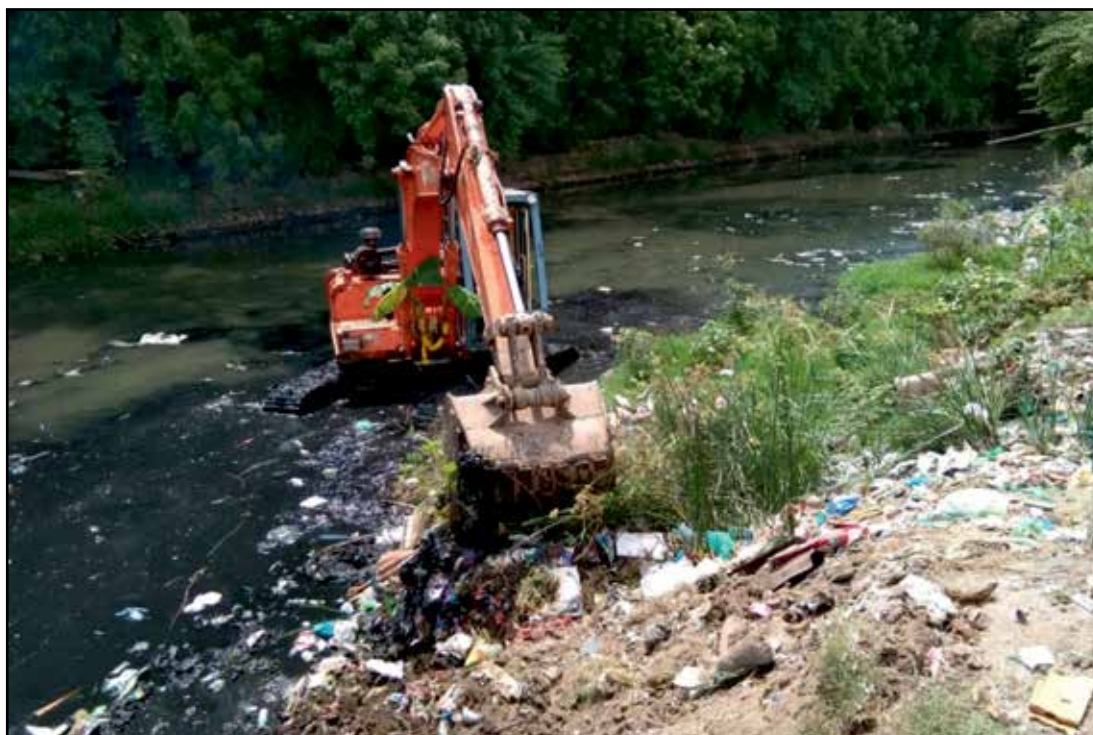
Desilting of Water Bodies - Uppanar Canal
