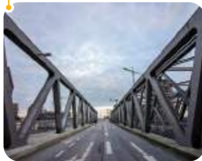
Structures for roads & bridges
