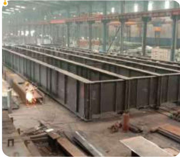
Gangapath : Patna Supply of Steel Composite Girders
