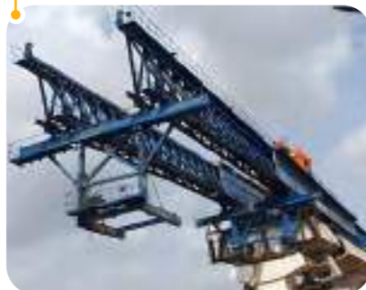
Launching girders for steel & concrete building structures
