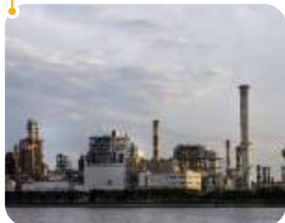
Primary & secondary structures for boilers & turbine generators
