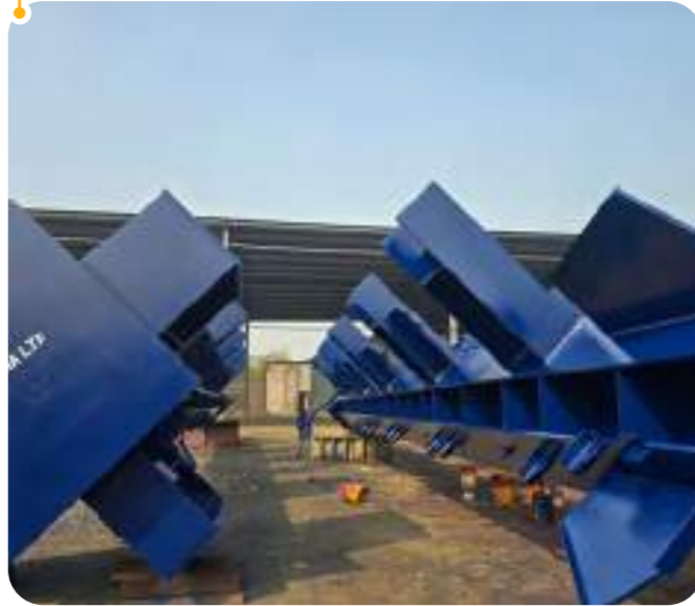
Arcelor Mittal Nippon Steel Expansion of Capacity Project
