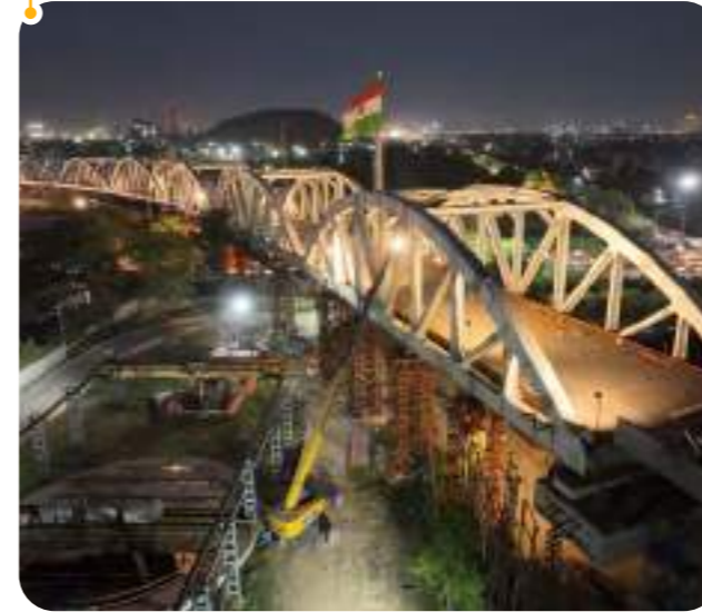
Rapid Rail Corridor between Ashoknagar and Barapullah
