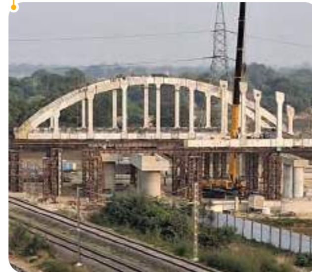
Bowstring bridge for Prayagraj City Road
