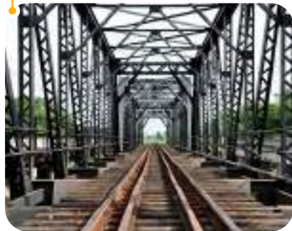
Railway's bridges & girders
