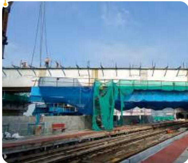
Chennai Metro Rail Corporation elevated Viaduct – Steel Spans
