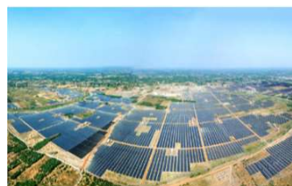
648 MW Ultra Mega Solar Power Plant
