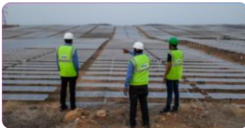
Conventional Module Cleaning System (Manual)
