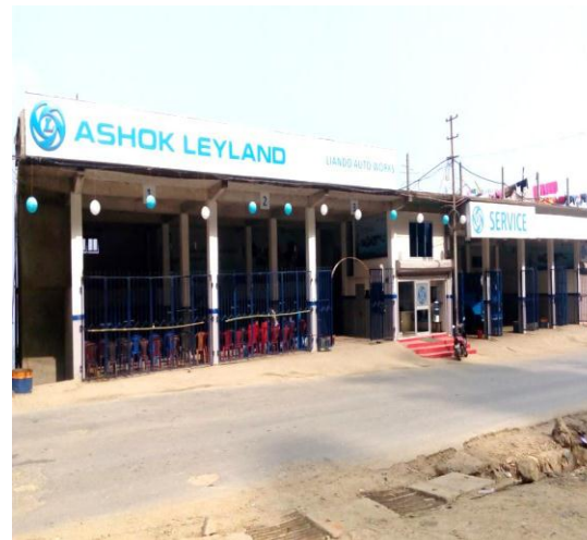
Authorised Service Center
