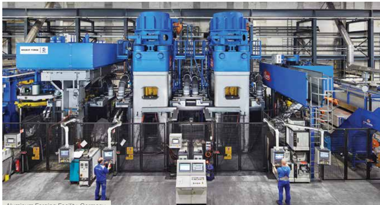
Aluminum Forging Facility, Germany
