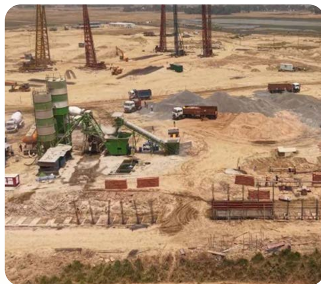
• Work under progress at Gorakhpur International Cricket Stadium
