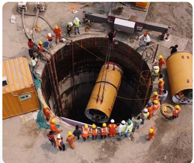
• Pipeline realignment using micro-tunneling technology at Beki river, Barpeta, Assam
