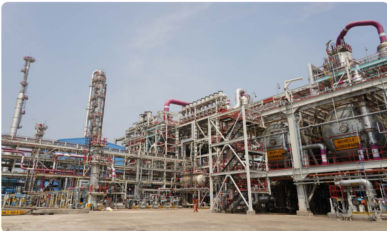
Butyl Acrylate Plant at Dumad, Gujarat Refinery
