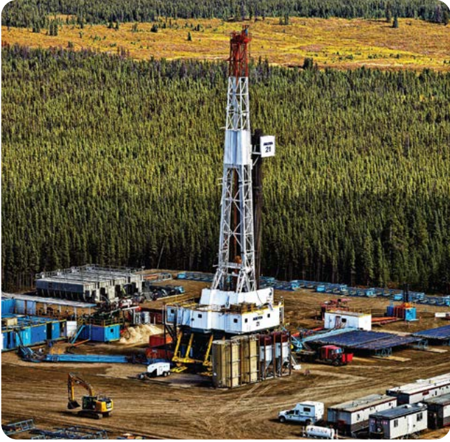
• Rig drilling operations at PNW Akita 21-042, Canada
