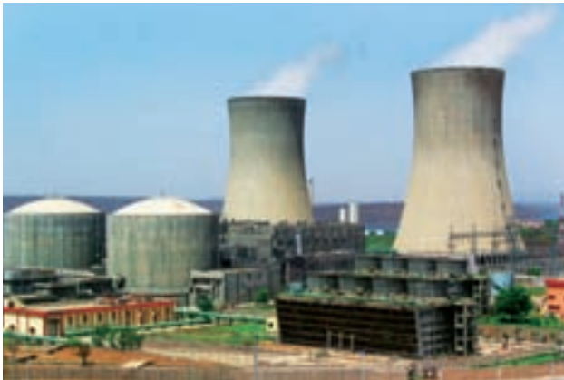
Natural draft cooling towers executed by L&T for Rajasthan Atomic Power Plant. L&T supplied critical equipment and built virtually every nuclear power plant in India.
