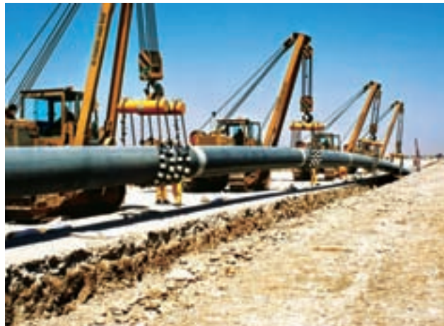
Lowering of 36" dia gas pipeline for Qatar Petroleum at Ras Laffan.
