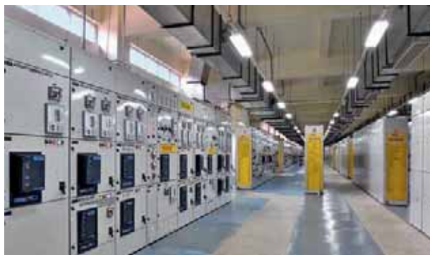
Switchboard installation at a power plant. L&T provides power distribution and control solutions – including LV and MV switchboards – across the value chain, from point of generation to end-user.
