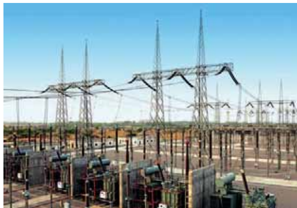
Substation incorporating 765 kV Air-Insulated Switchgear at Unnao in Uttar Pradesh. L&T offers complete solutions in high-voltage substations and power transmission lines.
