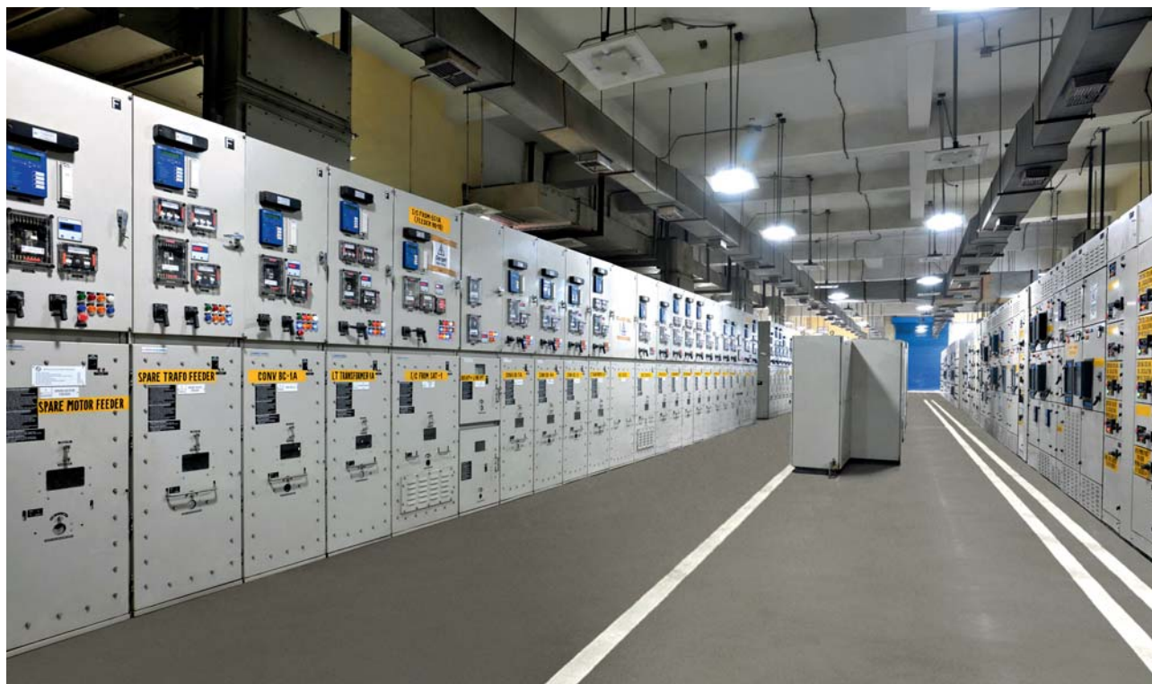
Switchboard installation at a power plant. L&T provides power distribution and control solutions across the value chain, from generation to end-user
