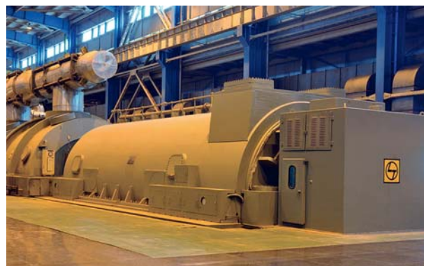
Enclosed turbine at a supercritical power project
