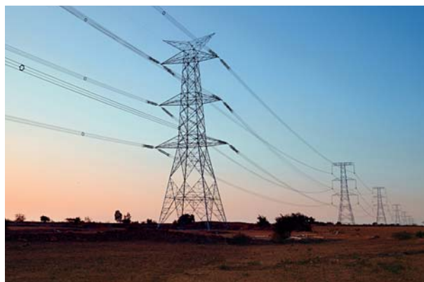
765 kV DC transmission lines at Kudgi, Karnataka
