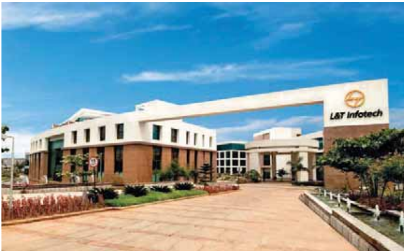
L&T Infotech's facility in Bengaluru.
