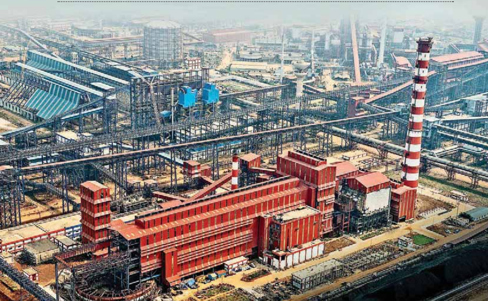
Integrated Steel Plant, Kalinganagar, Odisha.
