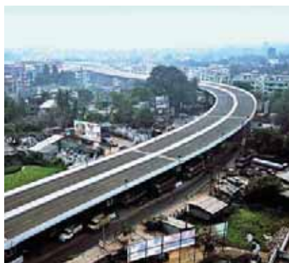
A flyover built by L&T.
