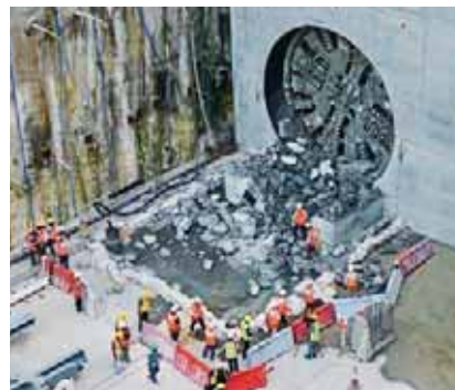
Tunnel-boring on the Doha Metro.
