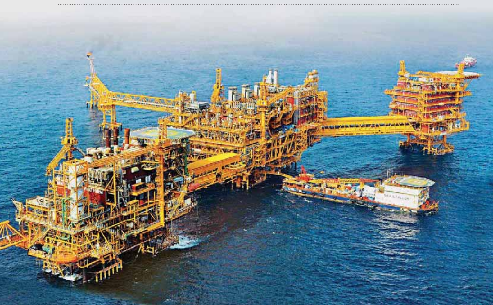
Mumbai High North (MHN) complex of ONGC, executed on EPCI basis. The massive complex comprises a process platform (26,500 MT topside + 13,500 MT jacket) a living quarters platform (6,500 MT topside + 13,500 MT jacket), two flare platforms and four bridges.
