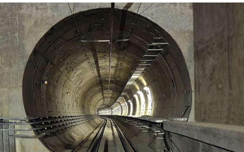
An underground section of the Chennai Metro.
