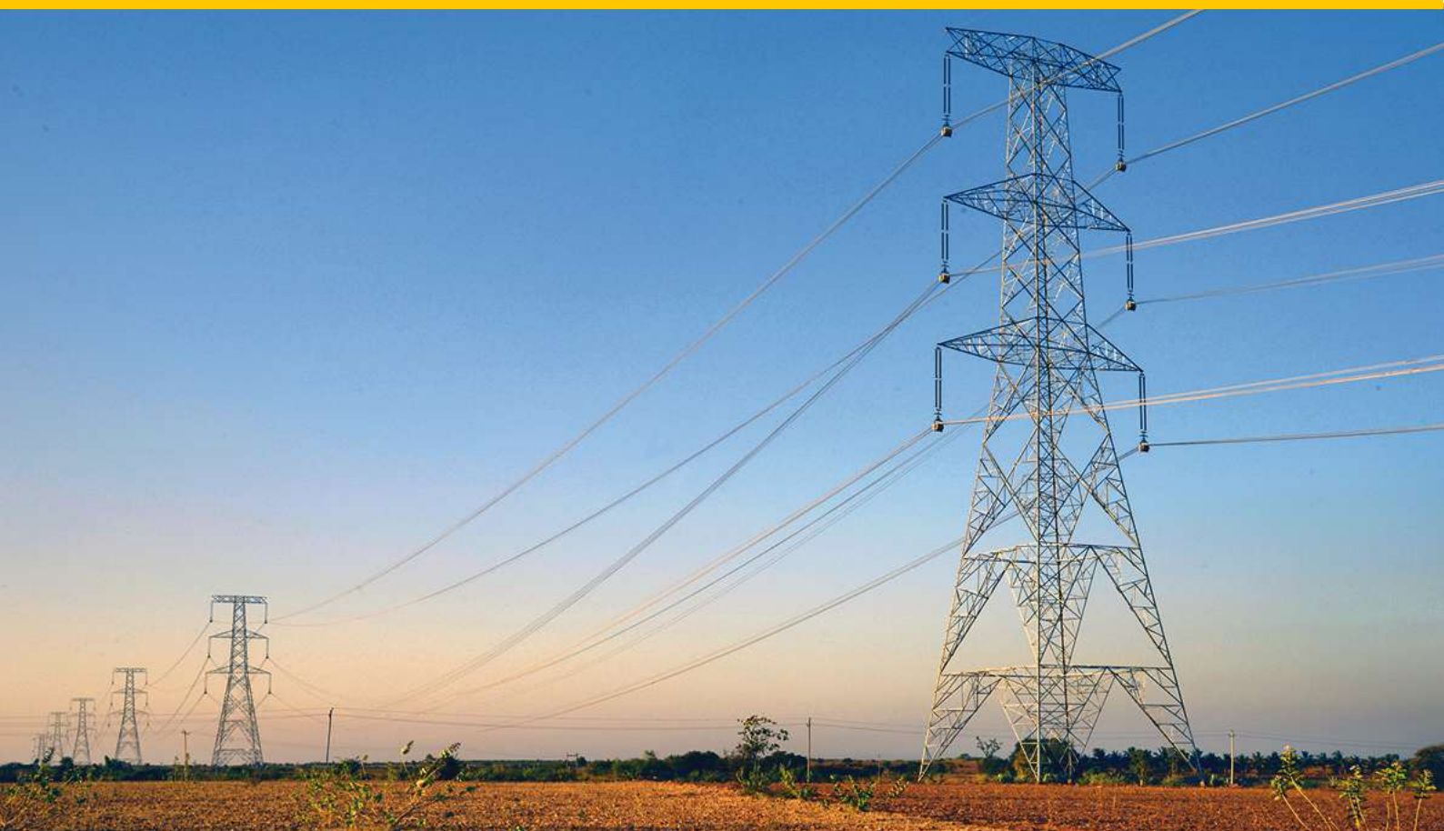
Kudgi Power Transmission Line project, Karnataka.
