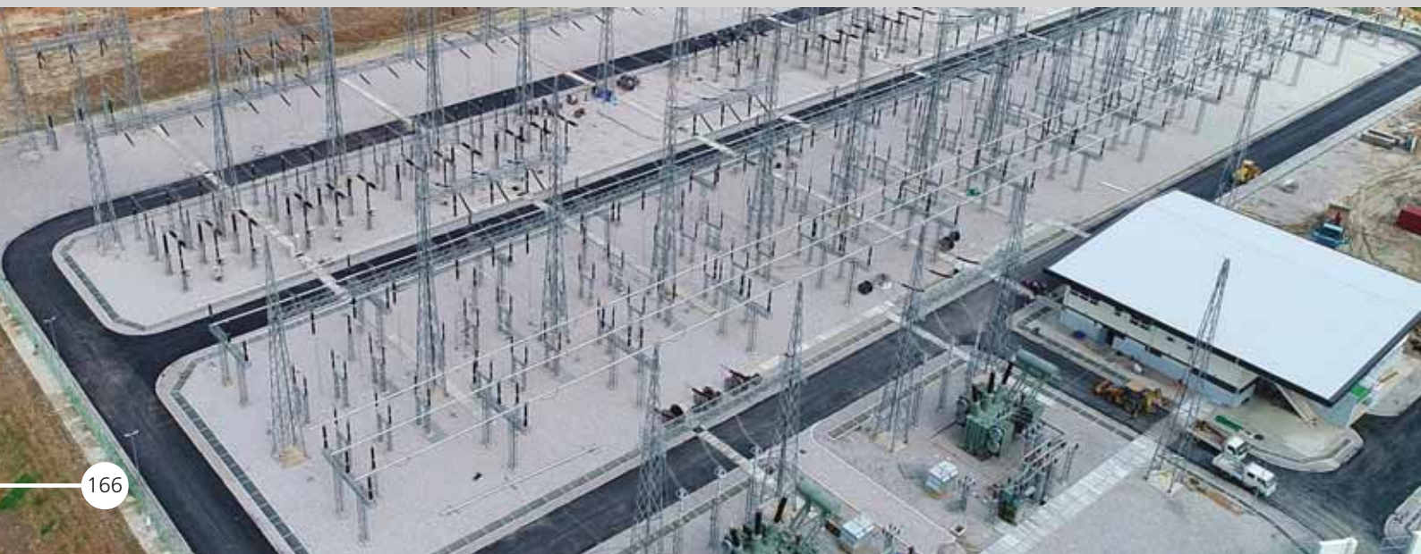
275 kV Air Insulated Substation at Lambir, Malaysia
