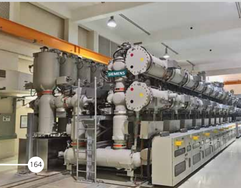
220 kV Gas Insulated Substation at Mehairja, Qatar
