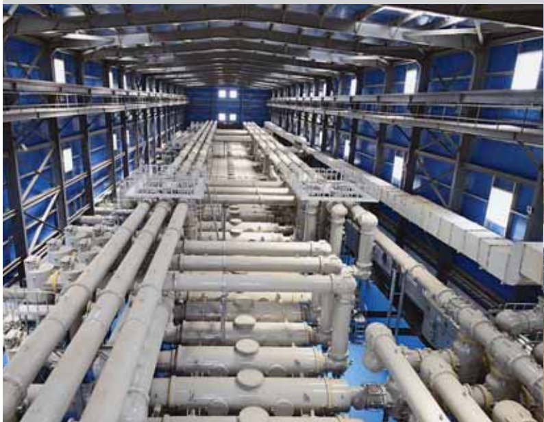
756 kV Gas Insulated Substation at Varanasi
