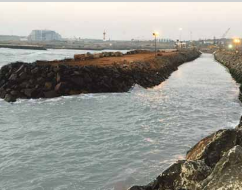
Break Water construction at Kudankulam Nuclear Project
