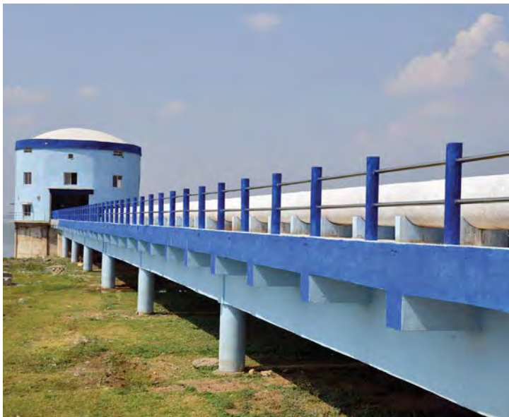
Medak and Sangareddy Water Supply Project
