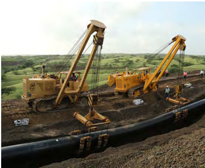
Laying of 36" x 67 km-long natural gas pipeline from Anjar to Mundra in Gujarat for Gujarat State Petronet Limited on EPC basis
