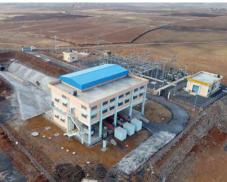
Pump house for Mohanpura Lift Irrigation Scheme
