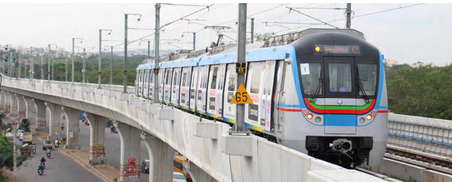
A section of the Hyderabad Metro
