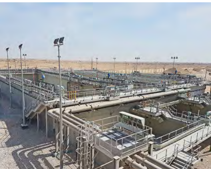
Al Shammal Water Treatment Plant at Qatar
