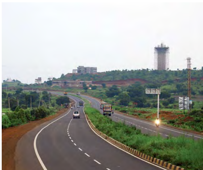
Solapur-Sangareddy Road Project
