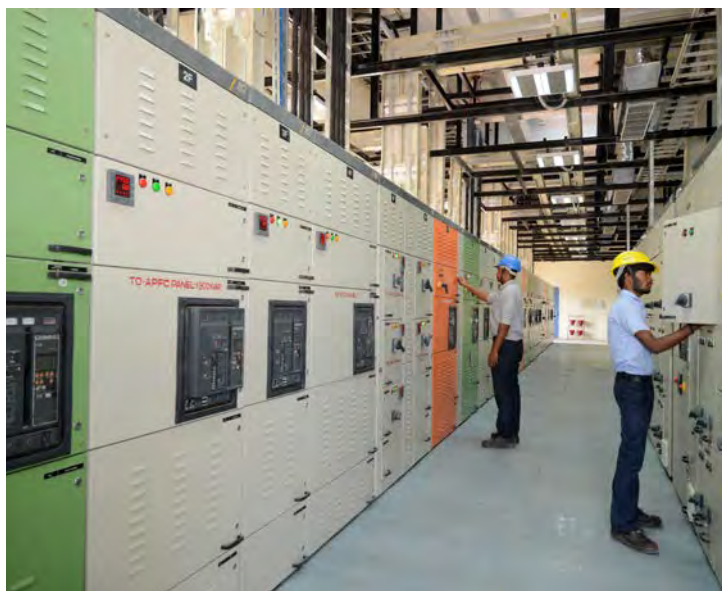
Switchboard installation at a national infrastructure site
