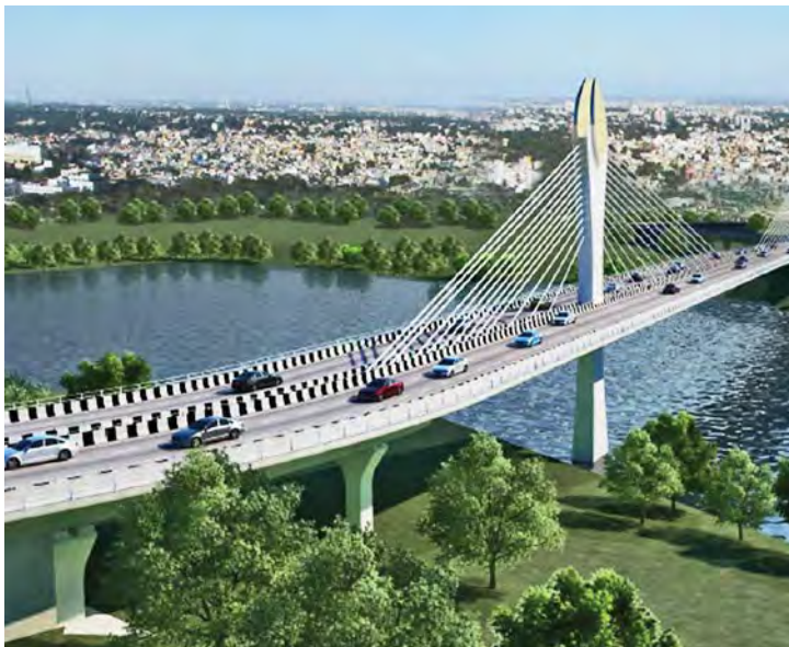
Cable-stayed bridge across Durgam Cheruvu Lake, Telangana
