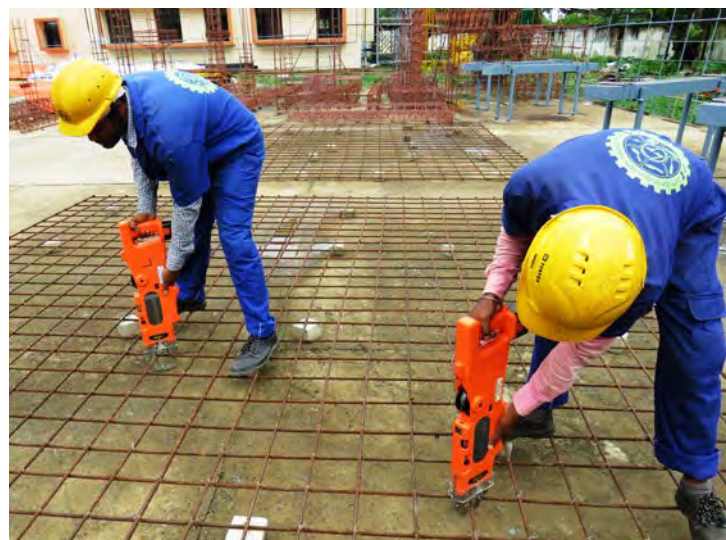
Training with Bar-tying machine, CSTI, Serampore, Hooghly, West Bengal
