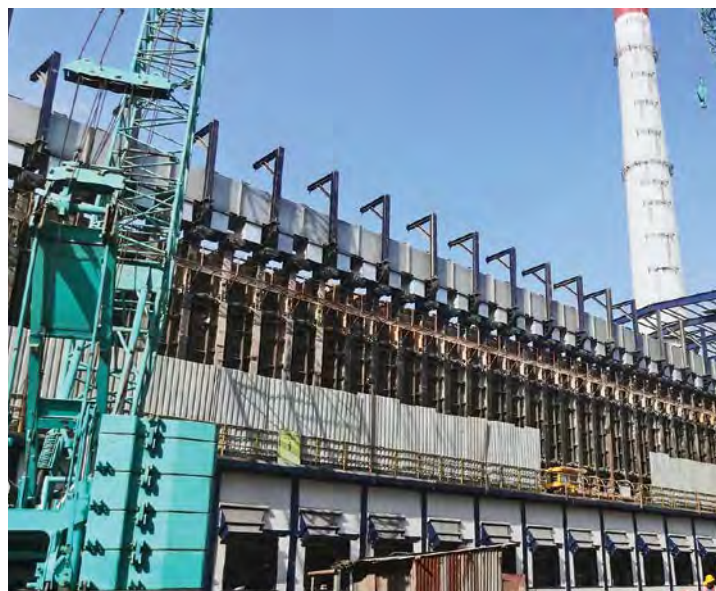
Coke Oven Battery
