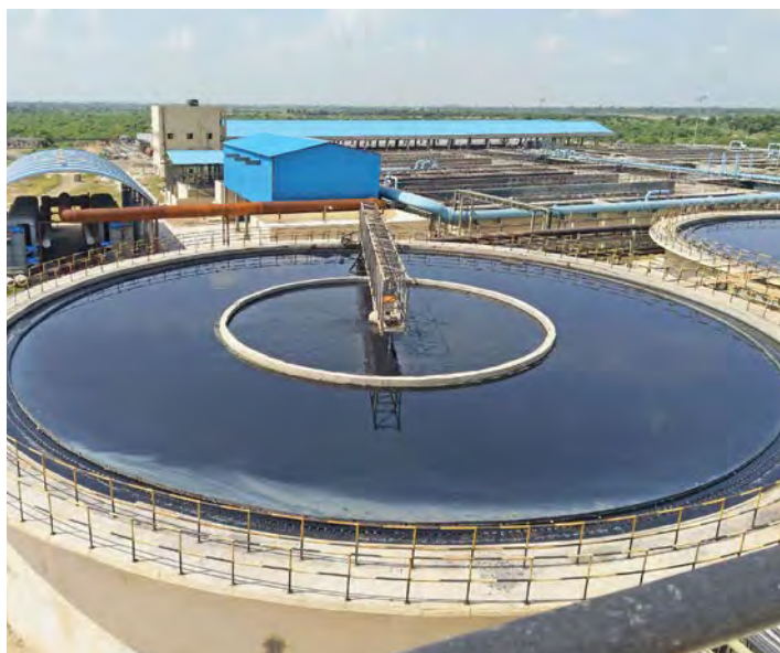
Common Effluent Treatment Plant, Narol
