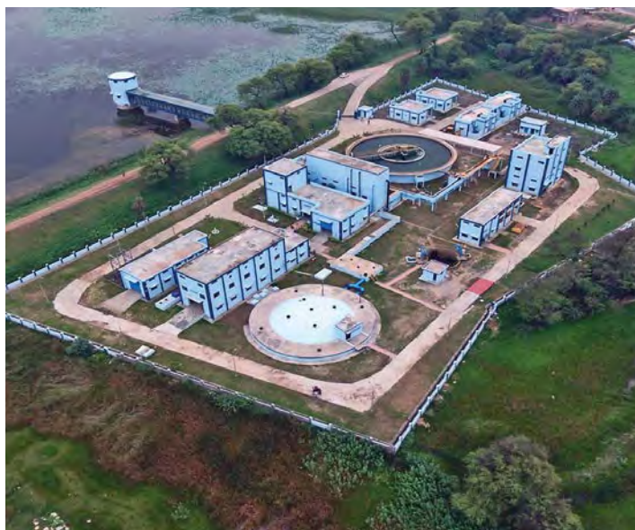
10.6 MLD Water Treatment Plant, Bagidora
