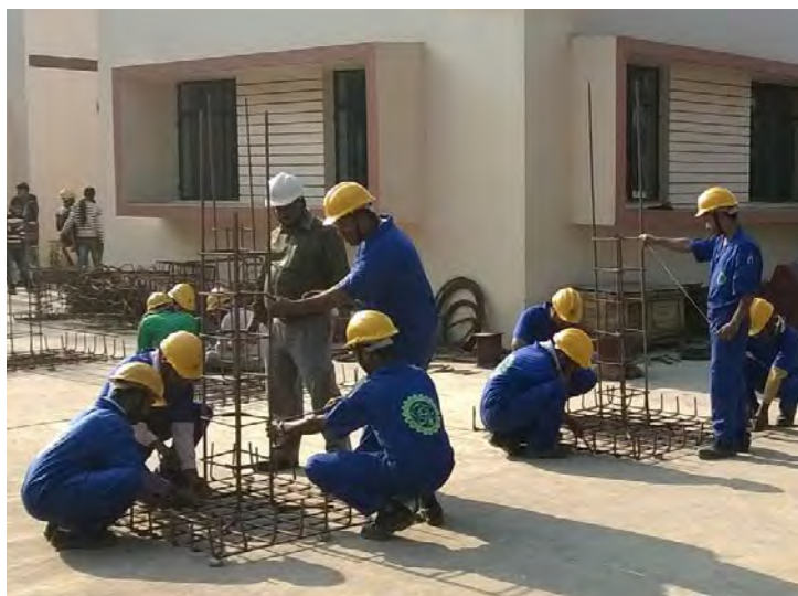
Bar Bending training in progress, CSTI, Serampore, Hooghly, West Bengal
