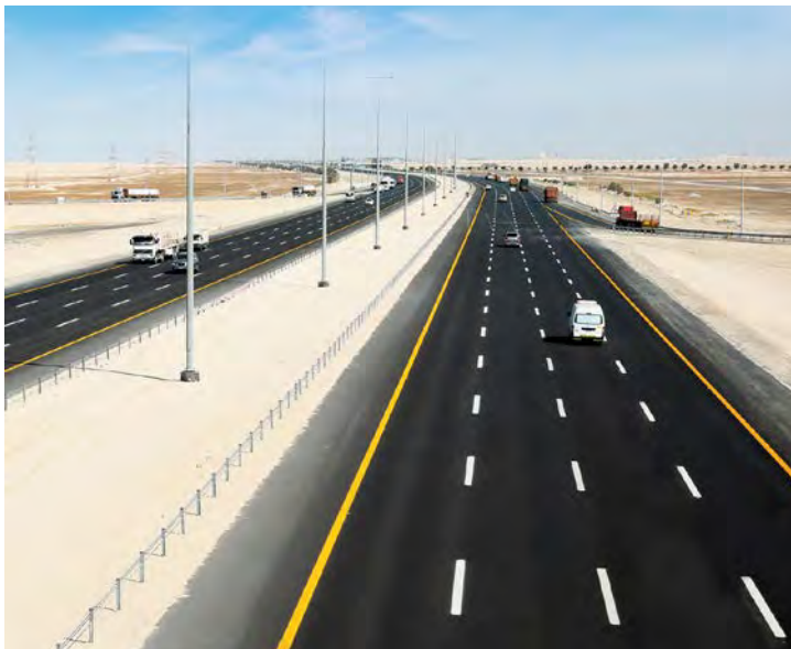
Mafrag-Ghweifat Highway, Abu Dhabi
