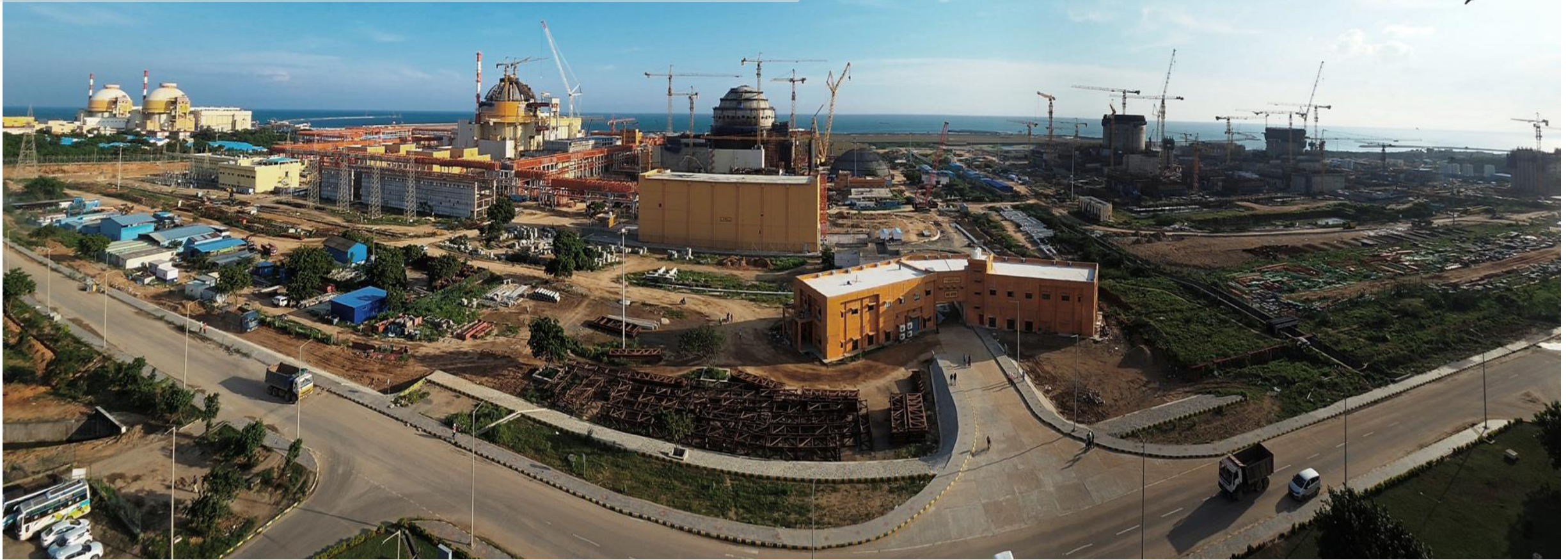
Kudankulam Nuclear Power Project
