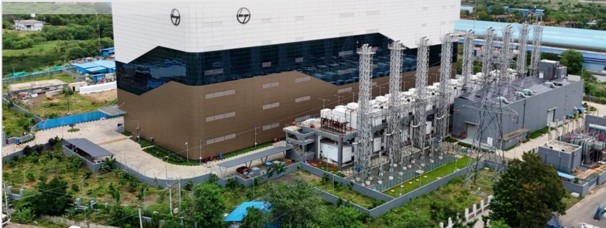
L&T Data Center, Sriperumbudur, Tamil Nadu
