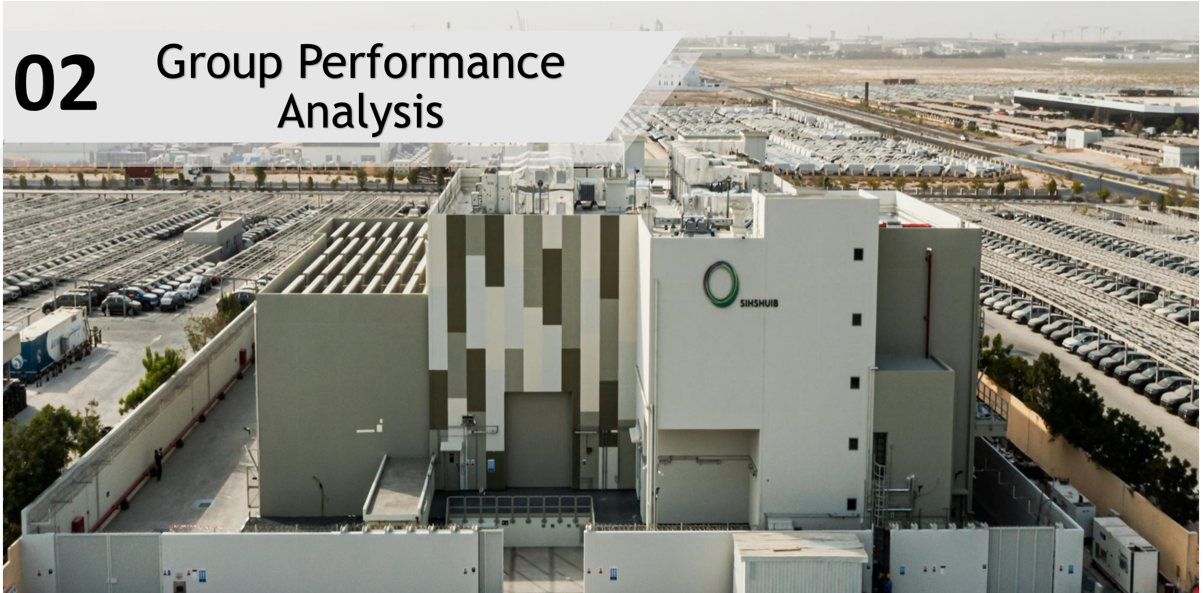
132/11 kV SIHSHUIB Substation – DEWA (UAE)
