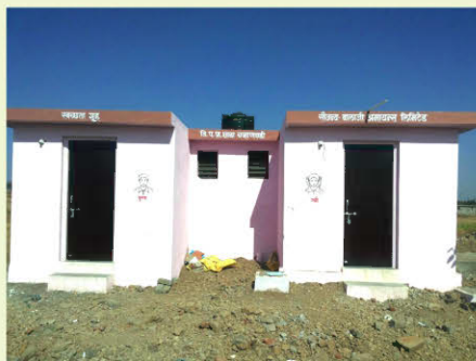
Toilet Blocks to Chawanwadi Village, Osmanabad District.
