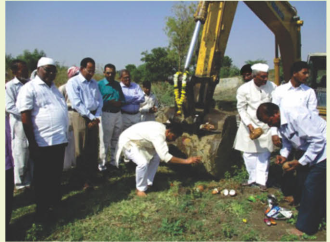
Channel Deeping Under Jala Yukth Shivar Abhiyan Tamalwadi Village, Osmanabad District.
