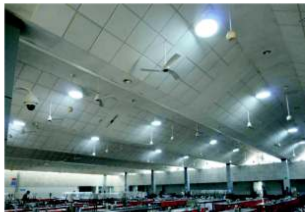
'Light Pipe' day lighting system in central complex canteen in Bangalore Plant.
