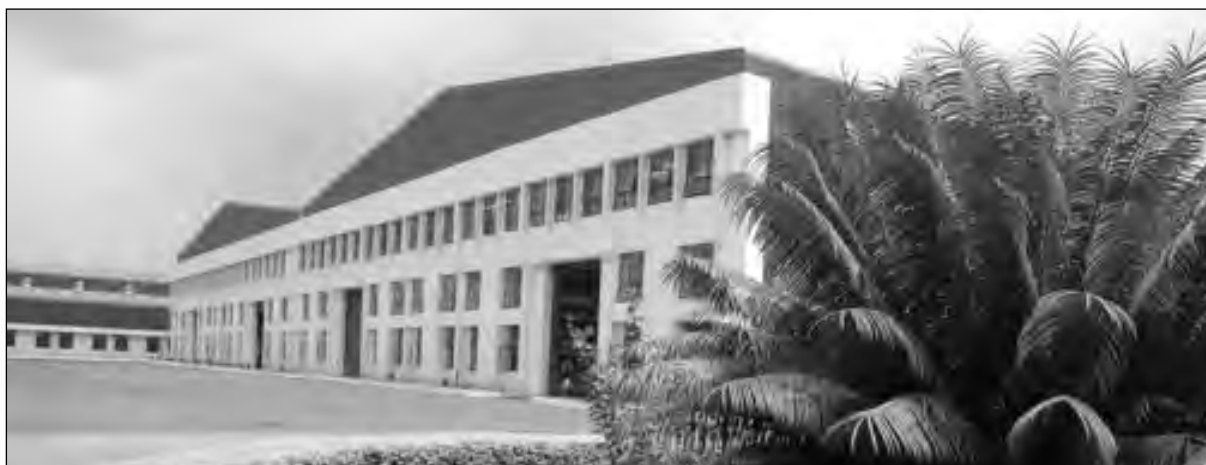
Premier's plant at Chinchwad, Pune
