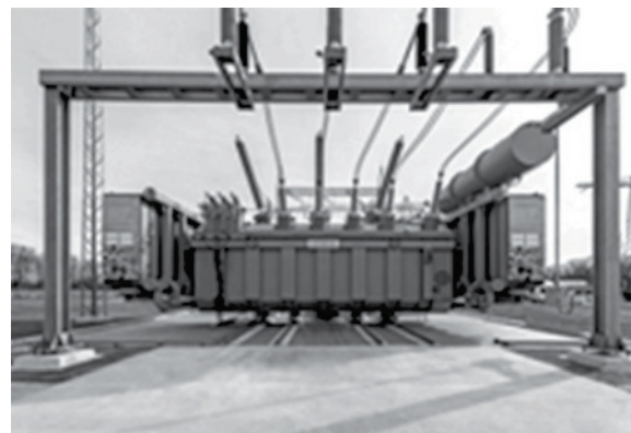
Ester filled Power Transformer
