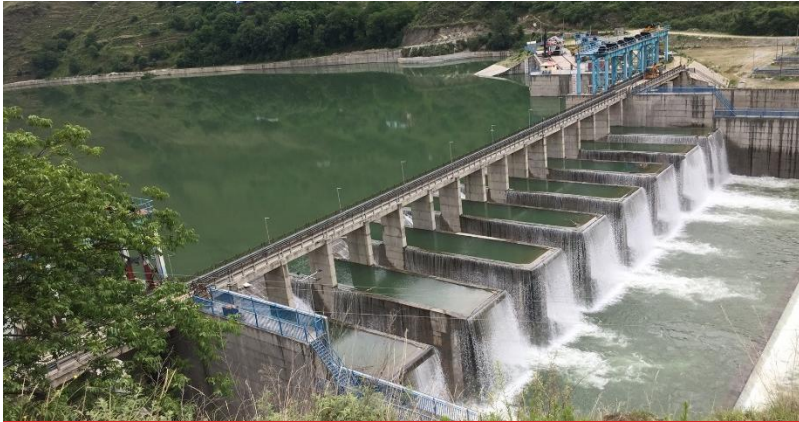
Sawrakuddu HE Project - Himachal Pradesh (111 MW) First Piano Key Weir in India
