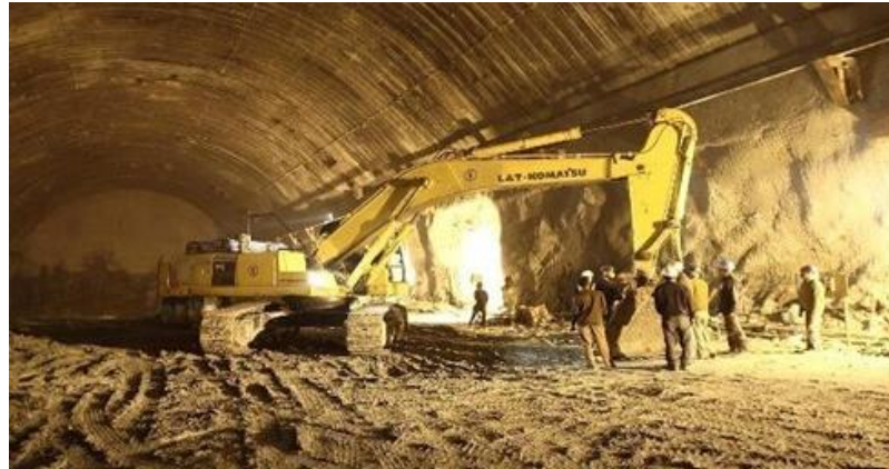
Srisailem HE Project - Andhra Pradesh (900 MW) Largest Underground Cavern in Asia 25.7m (W) x 53m (H) x 236m (L)
