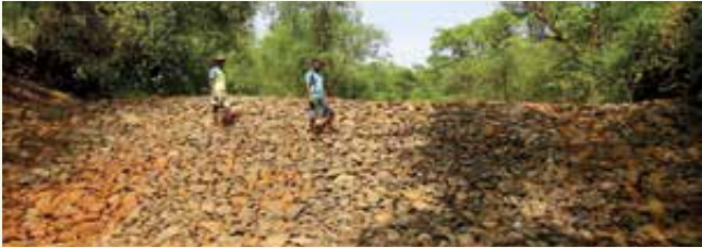
Loose boulder structure at Sakhar village, Khed, Ratnagiri
