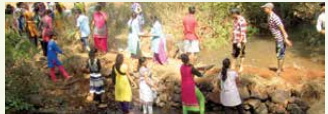
Vanarai Bandhara : A temporary barrier created for stopping flowing water and creating storage.
