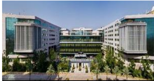
Embassy Qubix Pune (1.5 msf)
