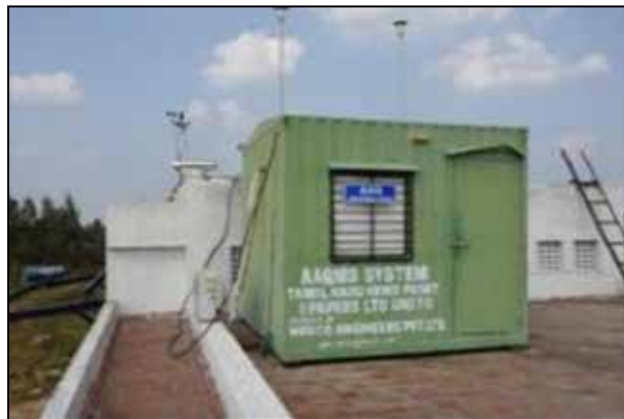
Continuous Ambient Air Quality Monitoring Stations
