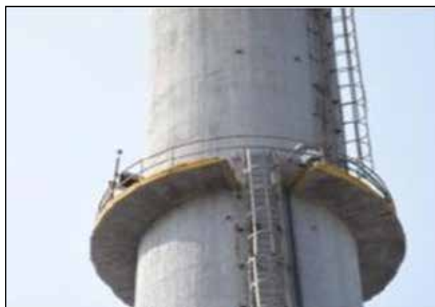
Continuous Stack Emission Monitoring Station
