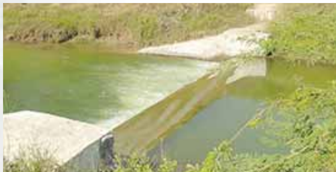
Construction of check-dams
