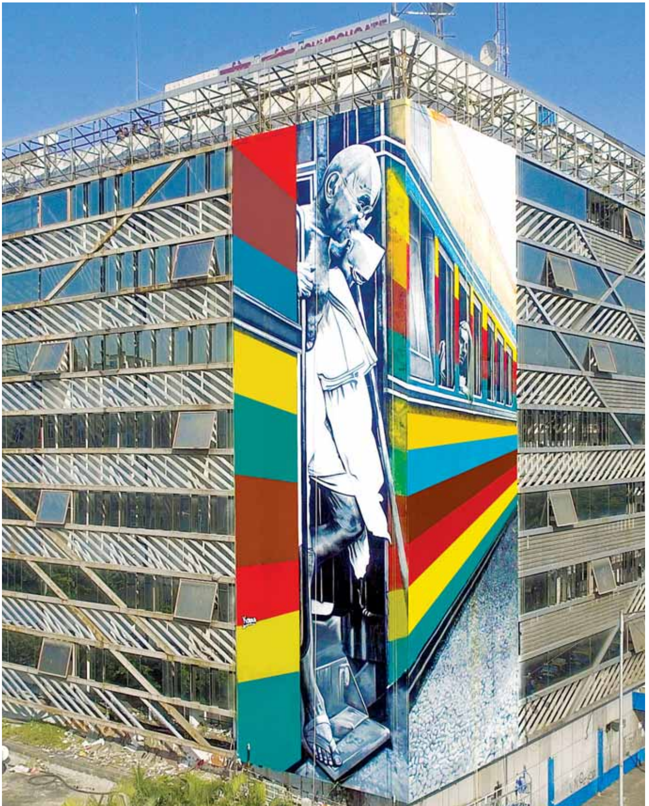
St+art India Foundation and Asian Paints, along with the gracious support of Western Railway and the Consulate General of Brazil came together to transform 'Churchgate station', one of Mumbai's busiest, into a work of art
