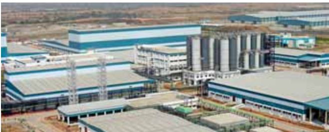
Paint manufacturing facility at Khandala, Maharashtra
