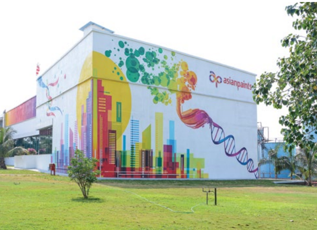
Research & Technology Centre at Turbhe, Navi Mumbai
