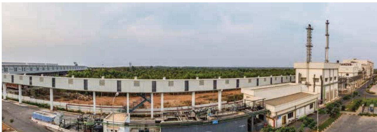
ITC's Integrated Consumer Goods Manufacturing Facility, Malur
