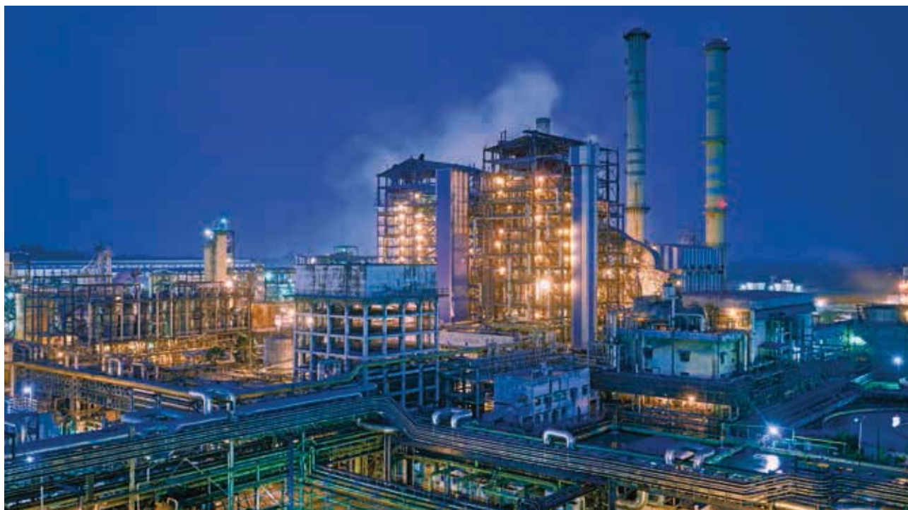
ITC's Paperboards Factory, Bhadrachalam
