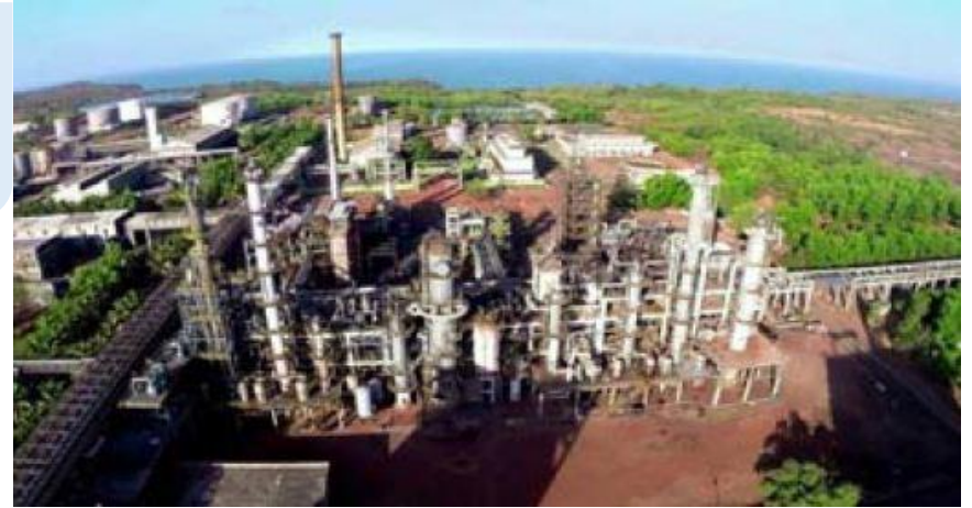
PVC resin Plant at Ratnagiri
