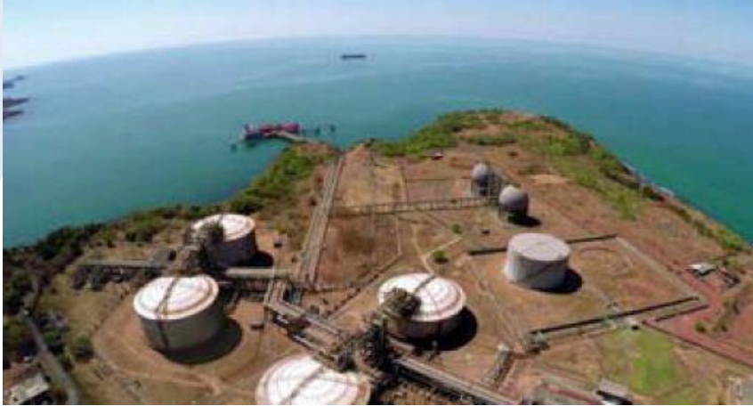
Storage tanks for raw material
