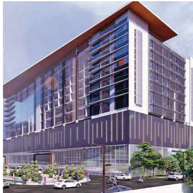
Vikrant Foundation, Saket
