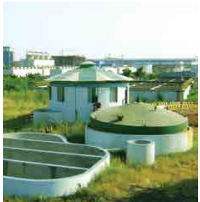
Bio gas plant
