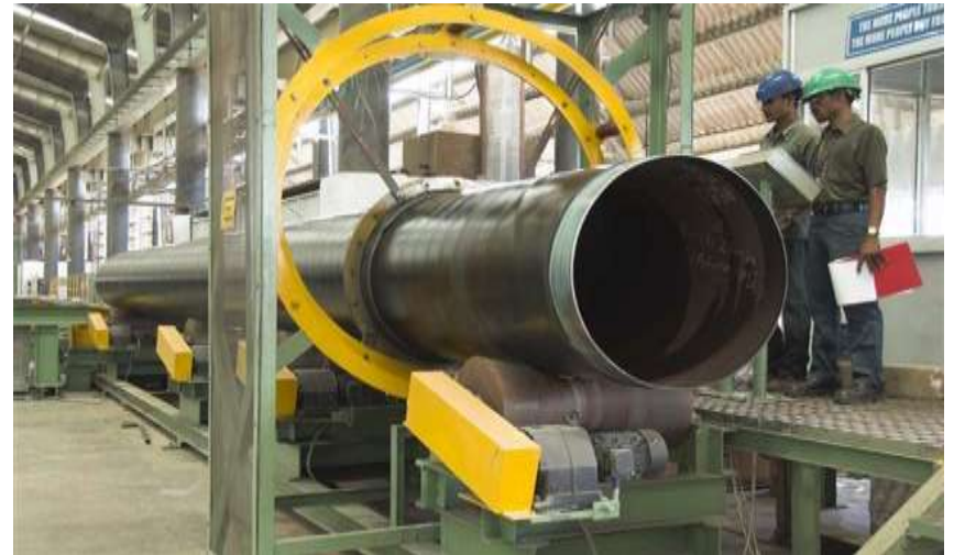
Pipe Coating – Anjar, US and Dammam
